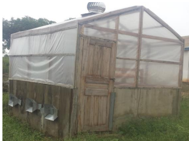
Figure 2: NSPRI solar tent dryer
